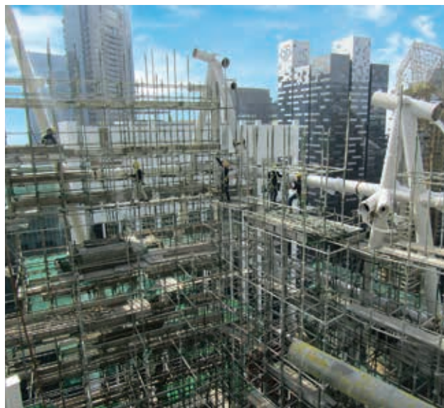
Roof crown installation works progressing (February 2018) – 18 Robinson
